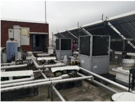
Fig. 1. Picture of the air source heat pump water heating system
