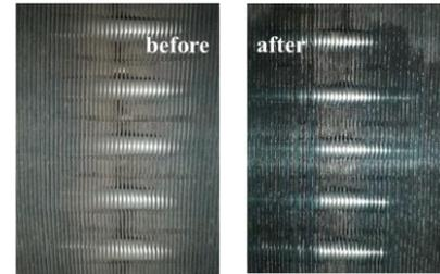
Fig. 9. The heat exchanger before and after cleaning
