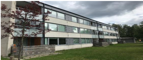
Fig. 1. South view of the case study building
